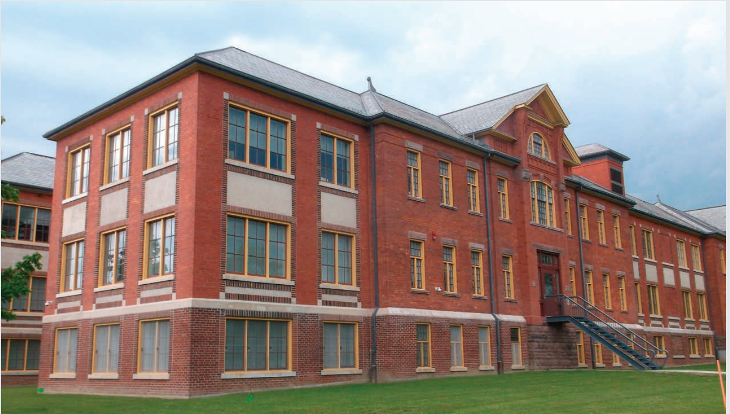
The buildings of the Asylum for the Insane in Mimico (now Toronto) designed by Kivas Tully and constructed between 1888 and 1894 have been adaptively reused as the Lakeshore Campus of Humber College. Photo Courtesy of Sharon Vattay
