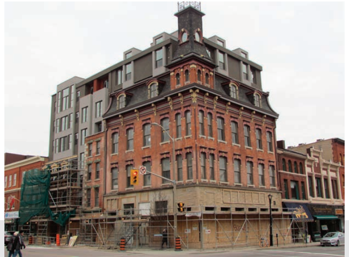
169-171 Wellington Street, Kingston, part of an adaptive reuse project, which will add residential units above the 1835 brick structure. Photo Lindi Pierce, 2017
