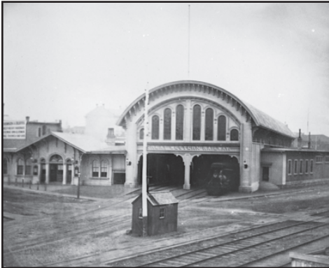
Great Western Railway Station (1864-5), Yonge St., northeast corner of Esplanade East, 1867. Photo Octavius Thompson, Courtesy of the Toronto Reference Library
