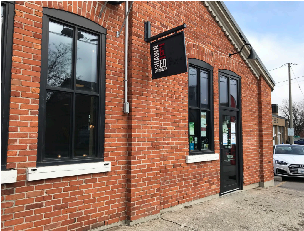
East section of the front façade showing the replacement steel windows with a two-over-two configuration replicating the original wood sash windows and the voussoir-arched brick lintels. The original window opening was enlarged to create the existing doorway. Below: Section of the east façade showing two bricked up openings, whose original use remains a mystery.
