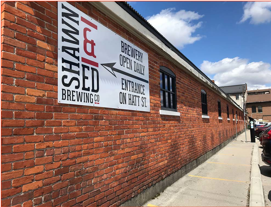
The long east façade of the building with eleven window bays.
