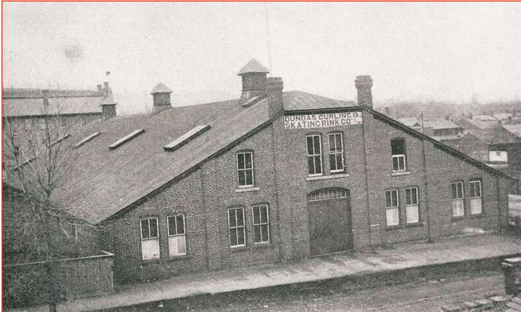
The Dundas Curling & Skating Rink, circa 1896. Photo shows the original façade with a single carriage entrance, and the original windows, four of the eight skylights and three square roof vents. ( Picturesque Dundas – 1972; reprint of original 1896 publication. (Dundas Museum & Archives: DM&A)
