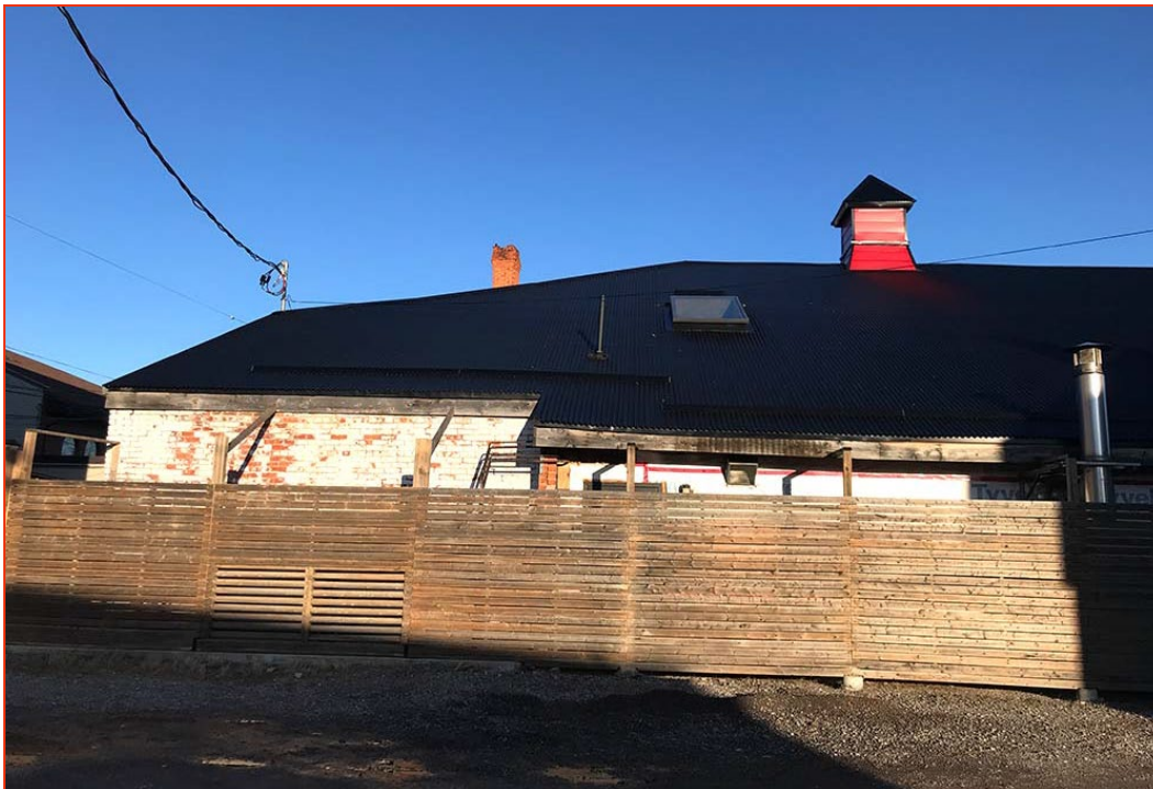
Rear section of west façade showing one of the four restored skylights and original roof vents, which are now only decorative elements as they are no longer needed for ventilation. View from parking area behind the former bowling alley building at 15 Foundry Street.
