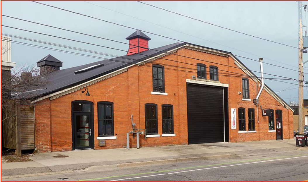
Front (south) façade of the Shawn & Ed Brewing Co. On the left is a new fire exit doorway and restricted access doorway for staff. The doorway at the east end serves as the entrance for customers. Truck deliveries are made through the rolling door entrance. (Chris/ Carol Priamo)
