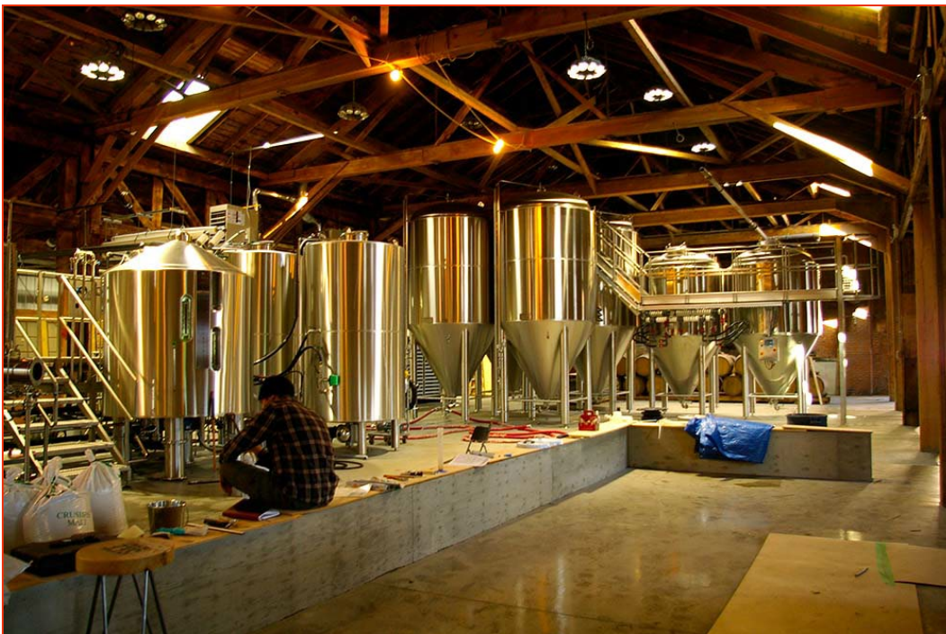
Renovations in progress, February 2016. View from entrance foyer looking towards the overhead rolling glazed door on the rear wall. Below: the production area with the stainless-steel tanks and the low wall separating it from the public seating area. Shows the timber roof framing and one of the four restored skylights.
