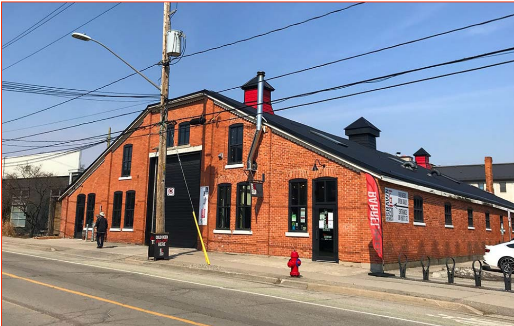
South and east facades showing two of the original roof vents (now closed) and a larger central one installed since 1981 (still functioning with two exhaust fans). The exhaust pipe was added when the wood-fired pizza oven was installed in 2021. All of the 2016-2022 photos below were taken by the author except where noted.
