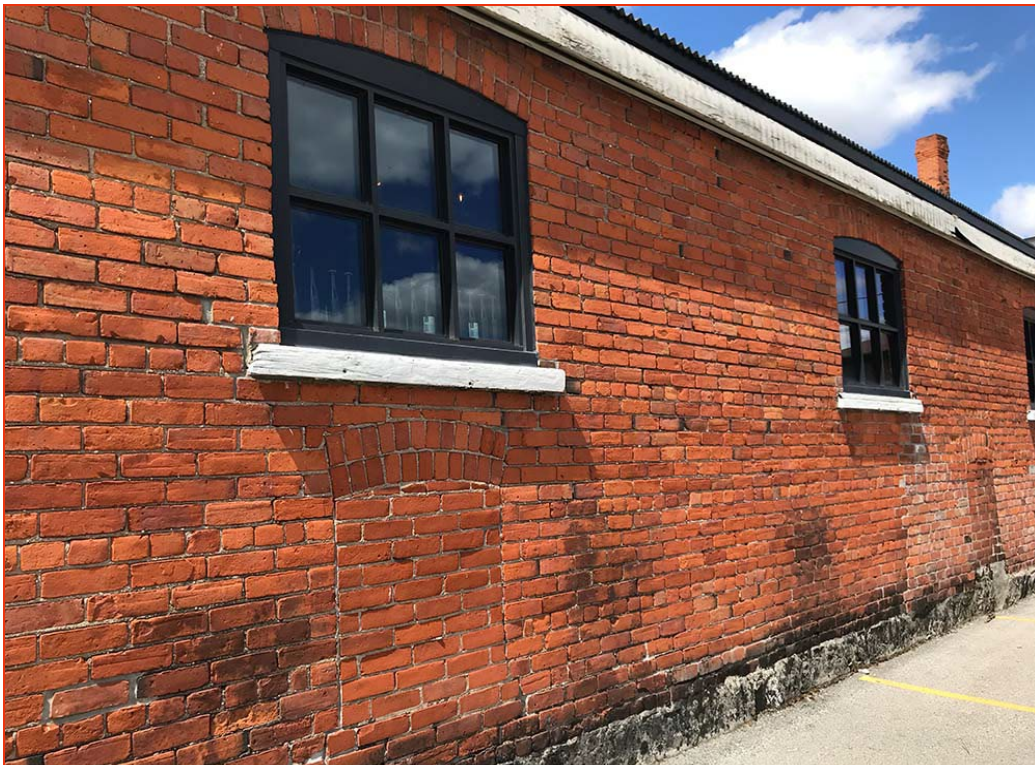
East section of the front façade showing the replacement steel windows with a two-over-two configuration replicating the original wood sash windows and the voussoir-arched brick lintels. The original window opening was enlarged to create the existing doorway. Below: Section of the east façade showing two bricked up openings, whose original use remains a mystery.
