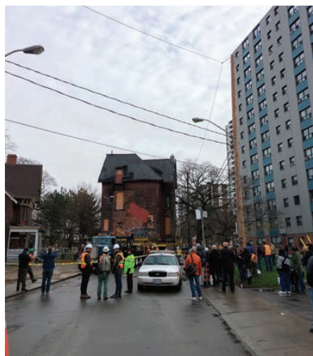
▲ The William Whitehead house relocation in November 2016. Photo Noah McGillivray, 2016
