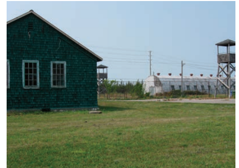
▲ Several of the 1940s structures, including hangars, were erected in haste during the war. Photo Lindi Pierce, 2014
