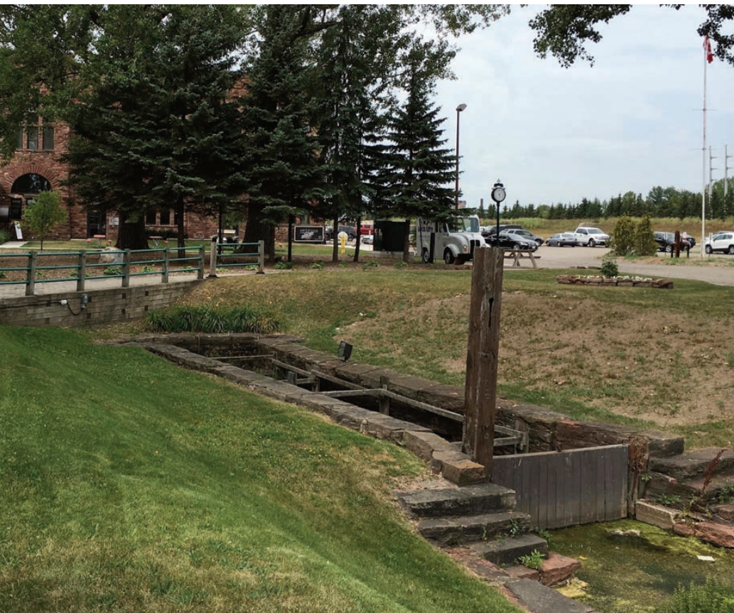
▲ The North West Company Canoe Lock in Sault Ste. Marie. Photo Chris Tossell, 2016.
