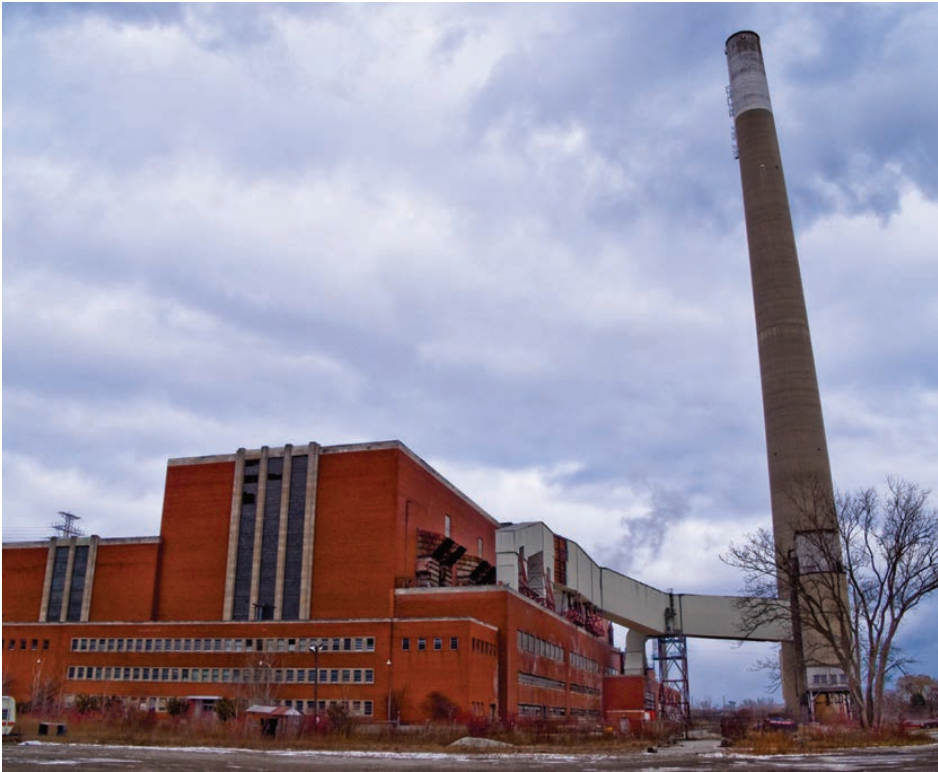
▲ Toronto's Richard L. Hearn Generating Station opened in 1951. Photo Richard Longley, 2017
