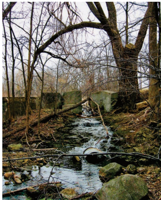
▲ Past the old car barns of the Sleeman street railway, Silver Creek disappears into a wooded area, trickling through the broken dam of a mill pond. Photo Susan Ratcliffe, 2006.
