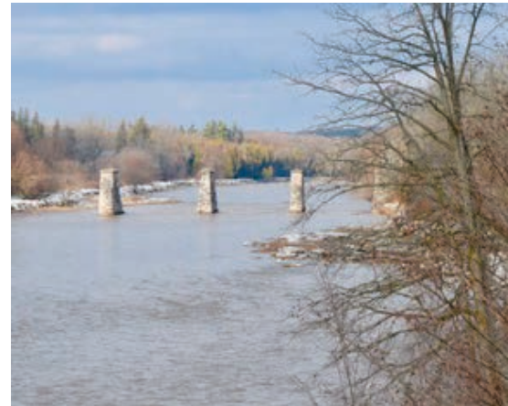
▲ Railway viaduct near Paris. Photo Dan Schneider, 2018
