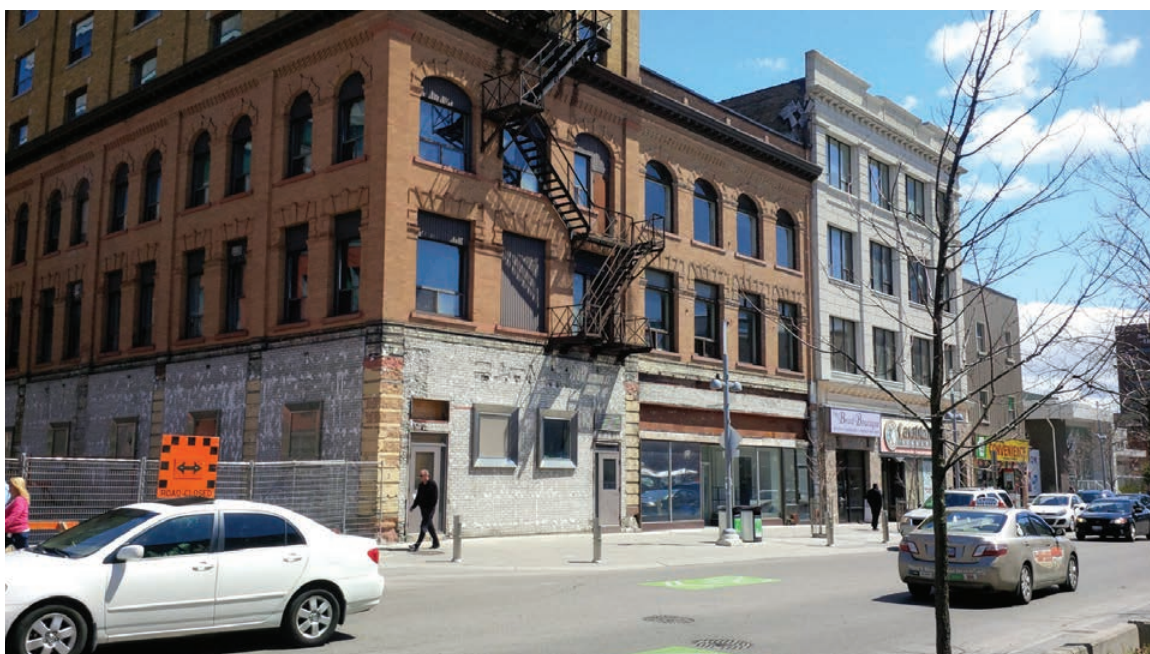
The Mayfair Hotel and Hymmen Hardware in April 2015, just before demolition. Photo Kae Elgie
