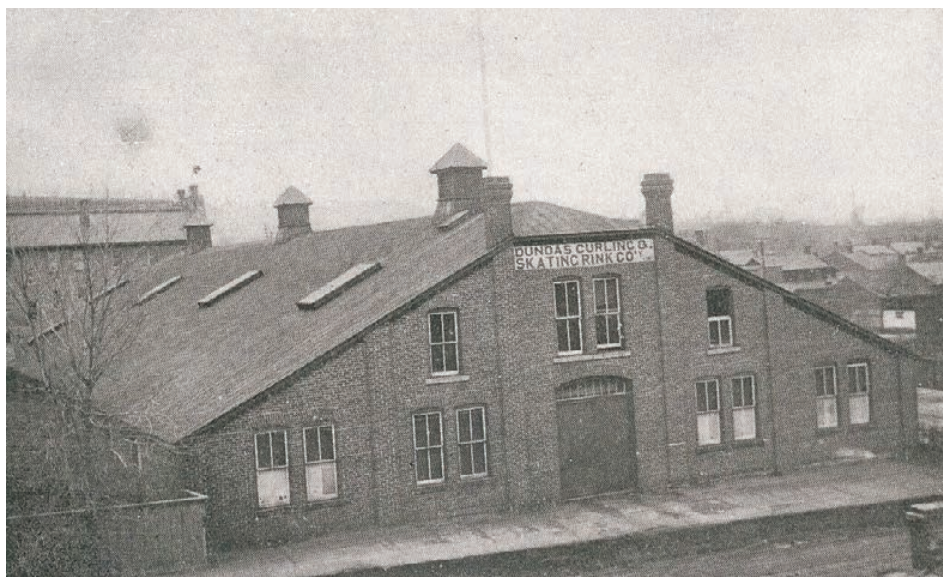
View of the front façade and roof section with original skylights (from Davidson and Pirie, eds., Picturesque Dundas, 1896). Photo courtesy of Dundas Museum and Archives
