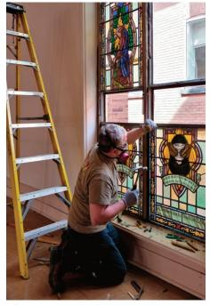
Wearing a respirator and protective gloves, Adam Frazee of Sunrise Stained Glass is using a hammer and chisel to free a section of one of the larger 1950s Luxfer windows.
