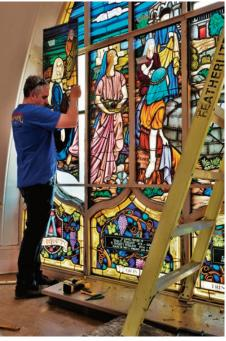
Adam Frazee lifting out one of the many panels that compose the 1994 window *I am the beginning and the end* by Joe Bullas of Bullas Glass, Kitchener.
