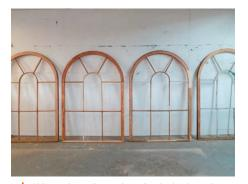
▲ Old growth wood was salvaged and spliced together with new wood using Dutchman repairs. **Photo** Em Cheng, 2016
